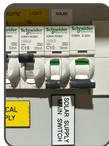
Example solar supply main switch
