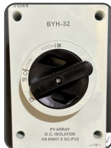
Example PV Array and DC isolator
