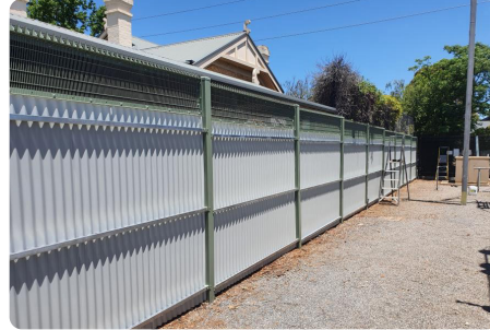
House and substation boundary fence
