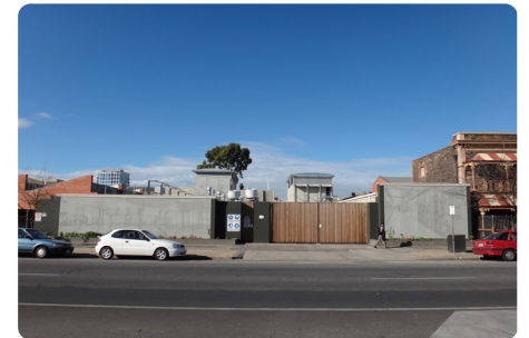
Substation blending into CBD areas
