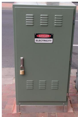
Figure 21: LV Switching Cubicle (above ground level)
