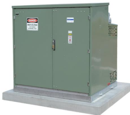
Figure 4: Typical Mk7 Transformer with 'Wilson Ring Main Unit'
