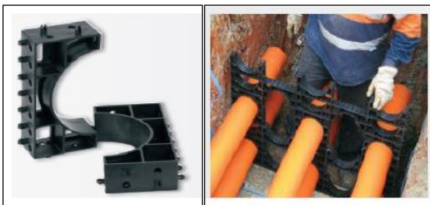
Figure 3: Example of Conduit Spacers
