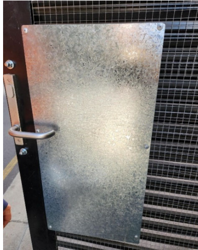
Figure 2 Security plate on internal handle
