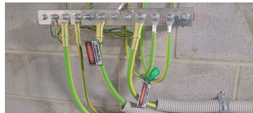
Figure 7: Multiple earth connection
