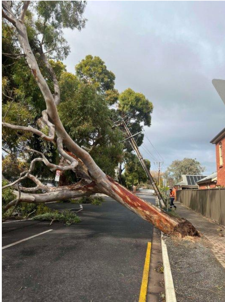
Figure 9: Fallen tree in metropolitan Adelaide brought down many spans of powerline.
